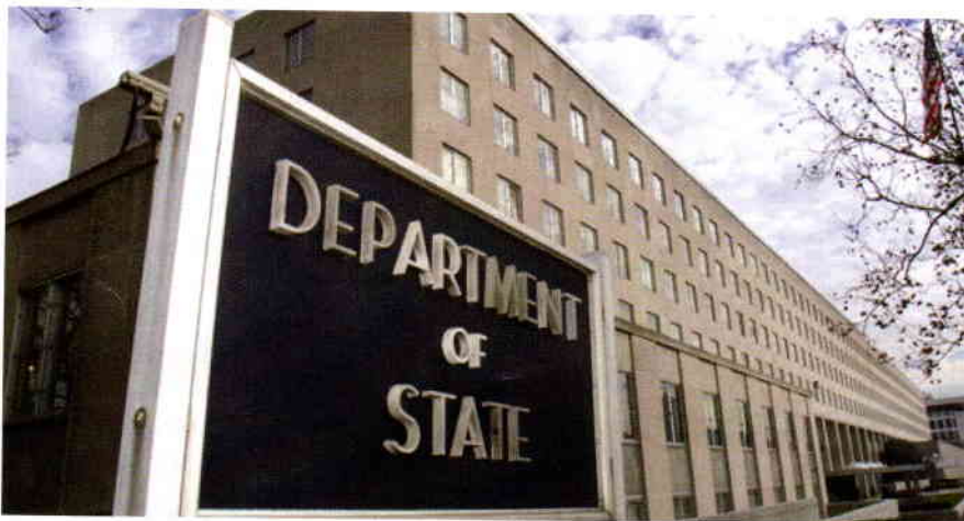
U.S. Department of State Headquarters Building, Washington, D.C.
